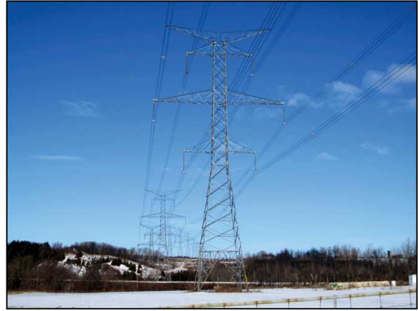
After New 500 kV Transmission Line
